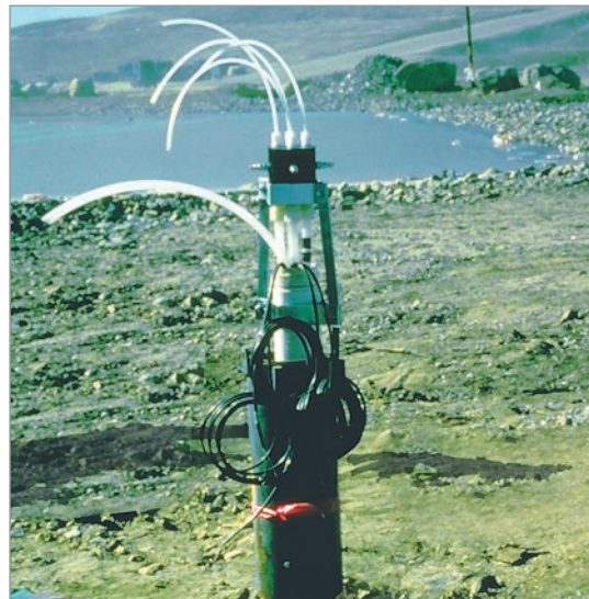
Landfill site over fractured granite, monitored with five Waterloo Systems. Each System comprised of dedicated Double Valve Pumps and Pressure Transducers in 4-6 intervals to depths of 275 feet (84 m). The Multi-Purge Manifold allowed the monitoring of 21 zones to be completed in less than 2 days.
